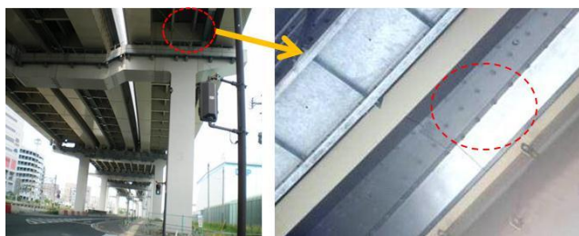
Fig. 2. Field test of monitoring caps at Kurosaki bypass in Kitakyushu-city from October 2010.
